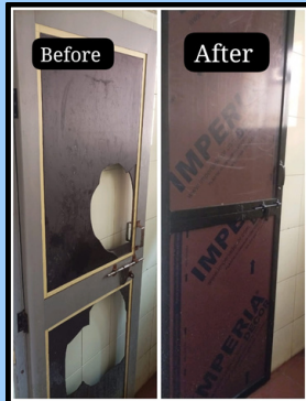
Renovation of washroom and distribution of Groceries, fruits at Snehangam school by RC Nagpur Green City
